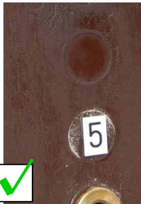
Fig. 11: OK Minor irregularities of surface and paint
